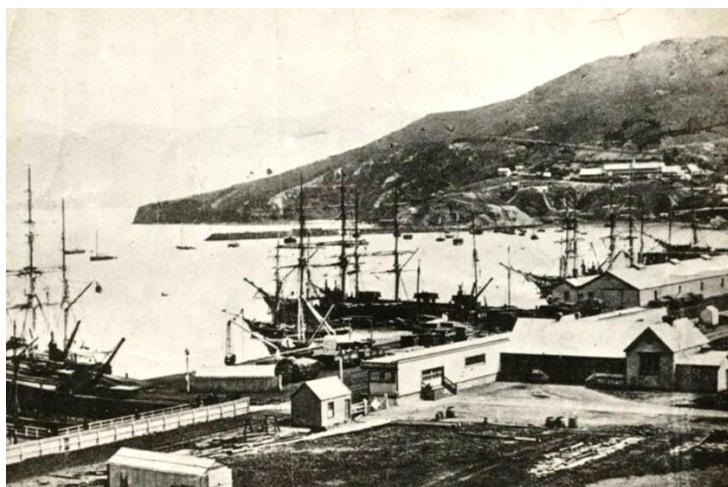
Lyttelton c. 1874. The first jetty, known as Thomas's or 'the Government Jetty,' was soon extended with the addition of screw piles.
