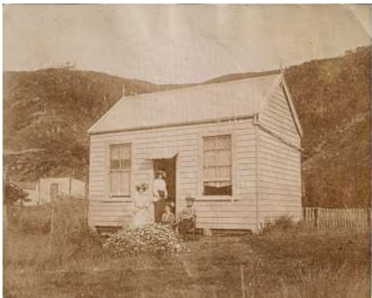
Before the verandah was added.
